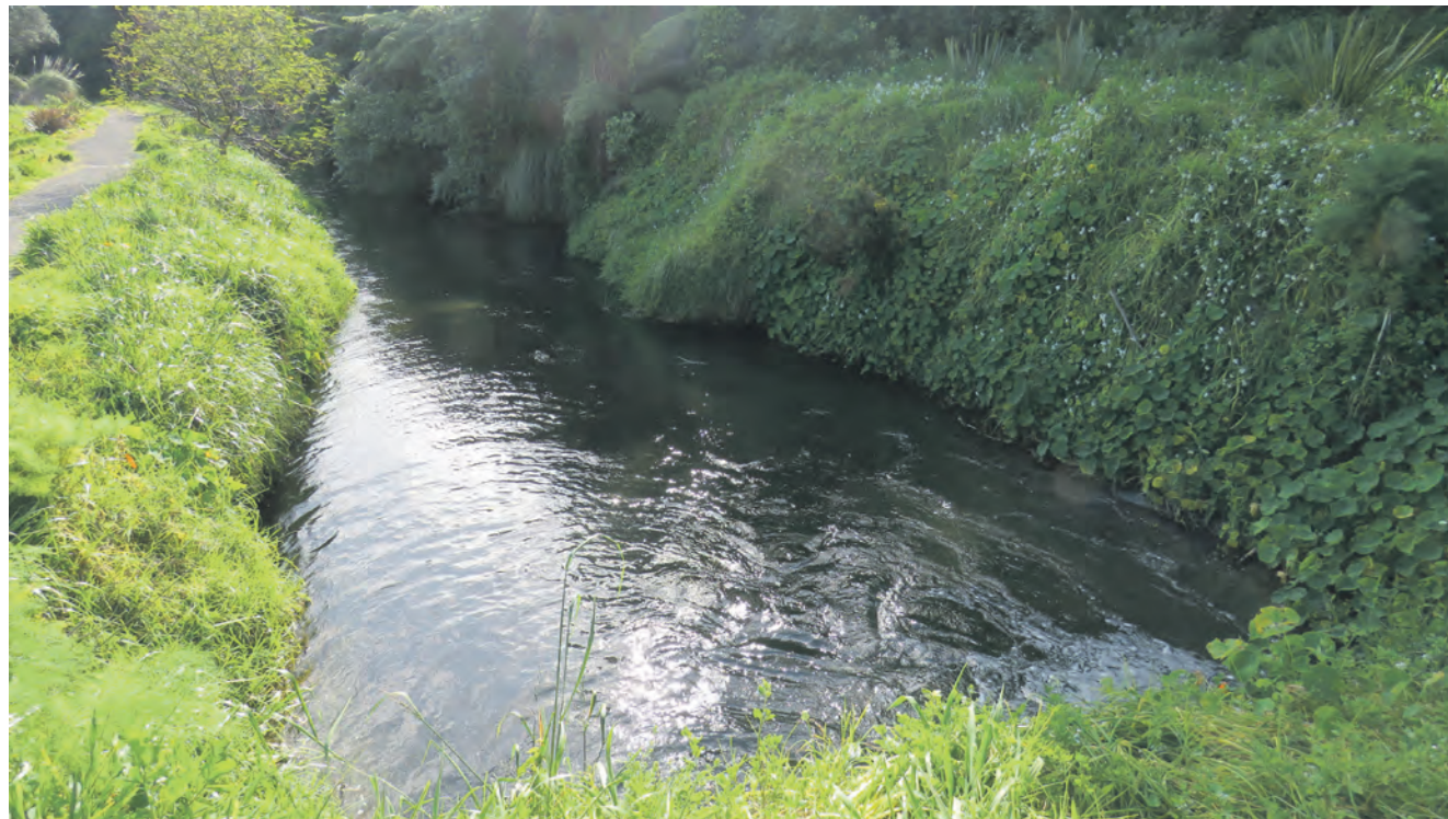
Water exiting the tunnel from the weir into the canal that leads to the lake.
